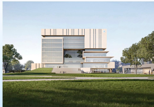
Zhejiang Vocational and Technical College of Transportation (Changxing Campus)
