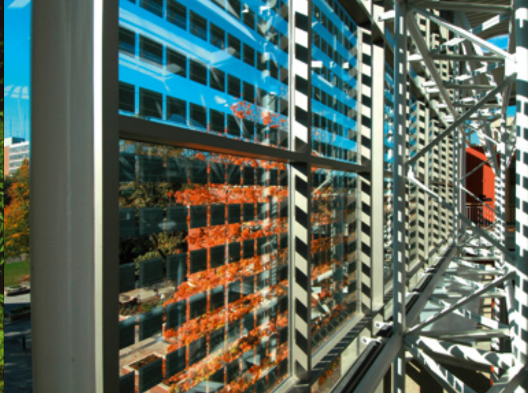
Milestone of building integration: This PV south façade of the university business school in Eugene, Oregon, was the largest vertical BIPV application in the U.S. at completion.
