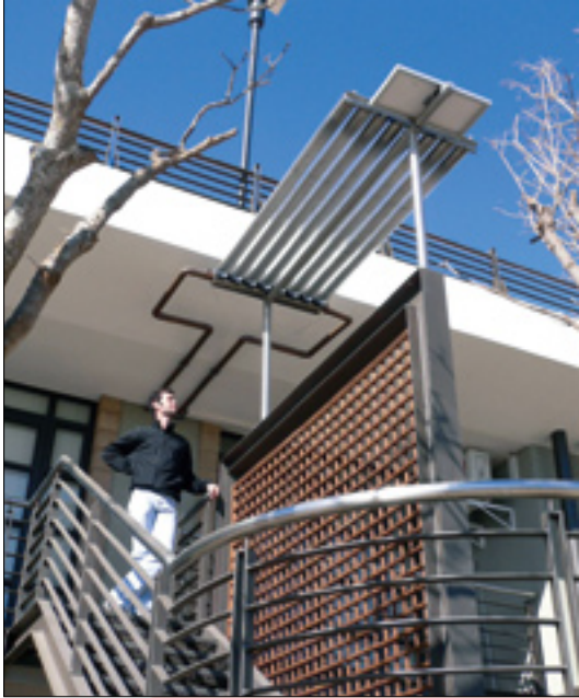
Smart architectural solution: solar shower with a vacuum tube collector planned by the South African company Omnibus Engineering
