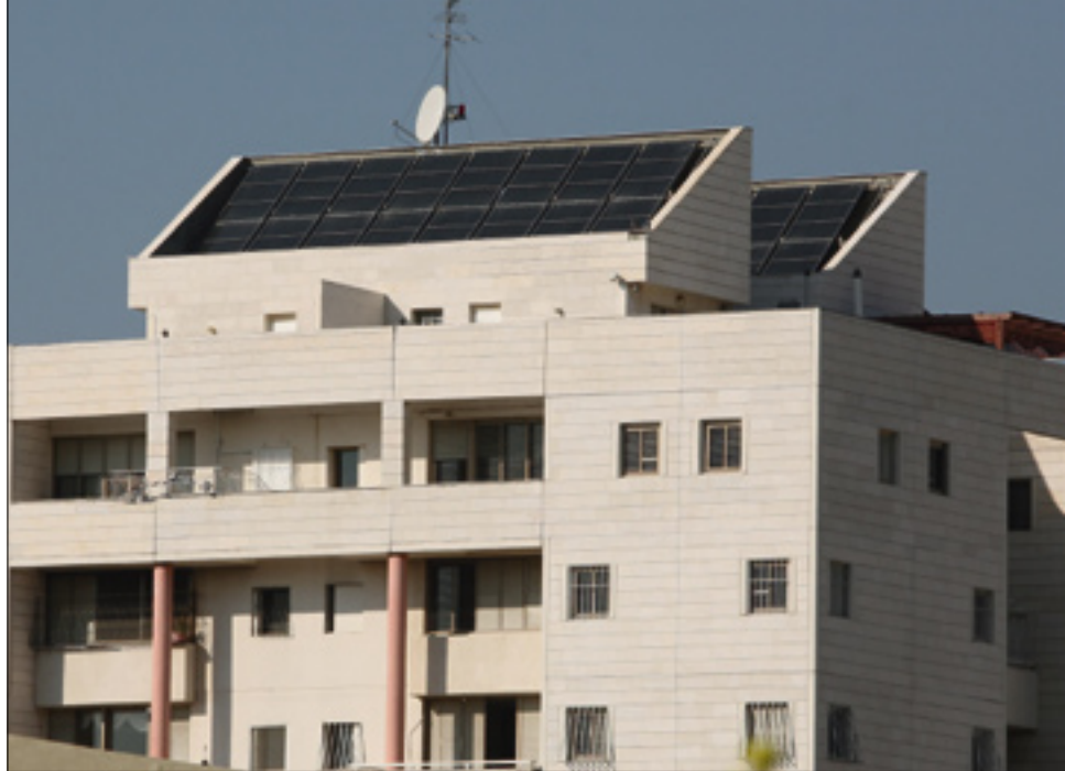
One way in which solar collectors can be architecturally integrated into apartment blocks.
