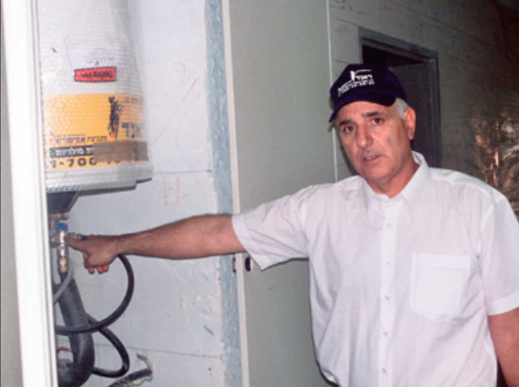
One tank per apartment: Eli Shilton from Rand explains the system technology of solar systems in high-rises.
